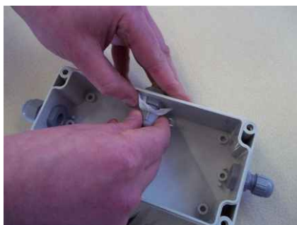
Step 7. Place nut over filter material and tighten
