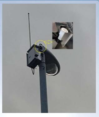
The Telensa system, as well controlling the lighting, can automatically pinpoint faulty lights. It gathers power consumption and other electrical information allowing energy consumption to be accurately measured.
